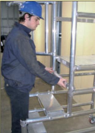
To work at the highest level fit platform on top rung and serrated climbing rung as shown.
