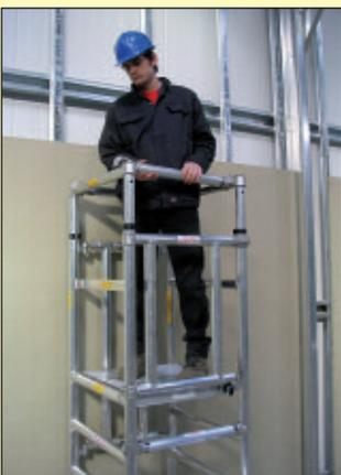
Horizontal braces complete the guard rail around the top working area.
