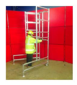
1) OPEN FRAME AND LOCK MECHANISM
