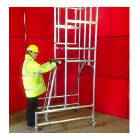
5) CLIP UPPER BRACE OF LADDER ABOVE RINGS ON VERTICALS WITH ASSEMBLED HOOKS ON TOP
